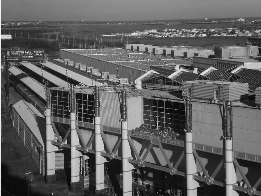
FIGURE 14.3 Rooftop solar array at the Atlantic City Convention Center.
