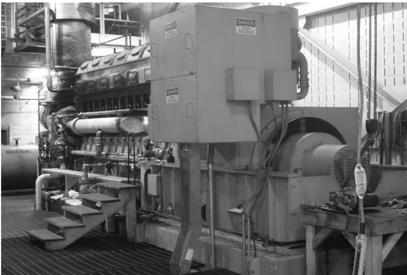
FIGURE 6.3 Genset using landfill gas in Johnson City, Tennessee.
