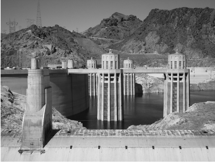
FIGURE 4.2 Low water levels of the reservoir at the Hoover Dam in 2010 reduced plant electrical output.
