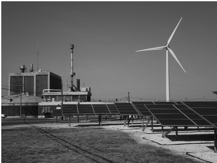
FIGURE 8.3 Hybrid wind and solar PV generation for the Atlantic City wastewater plant.
