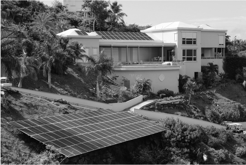
FIGURE 3.7 Residence using solar PV on St. Thomas Island, U.S. Virgin Islands.
